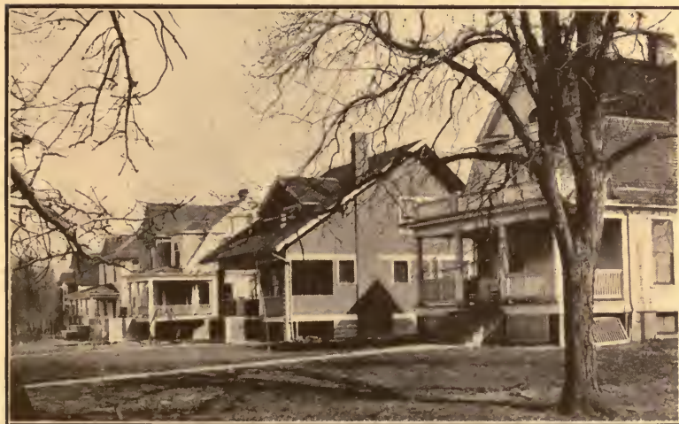
VIEW ON EAST MAIN STREET, BENTON
